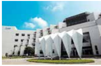
Tainan Plant (Diamond-rated Green Building)
